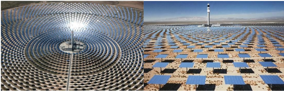
Figure 27. Concentrated solar power (CSP) mirrors laid out with phyllotactic geometry to optimize energy generation (Source: Pawlyn, 2019)
