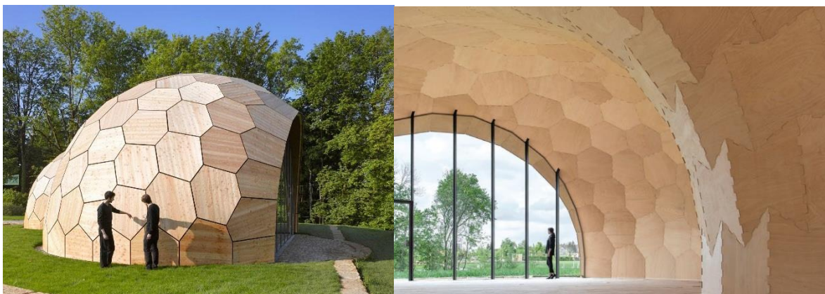
Figure 6. Landesgartenschau Exhibition Hall at the University of Stuttgart – Based on the Structure of a Sea Urchin Skeleton (Source: Pawlyn, 2019)
