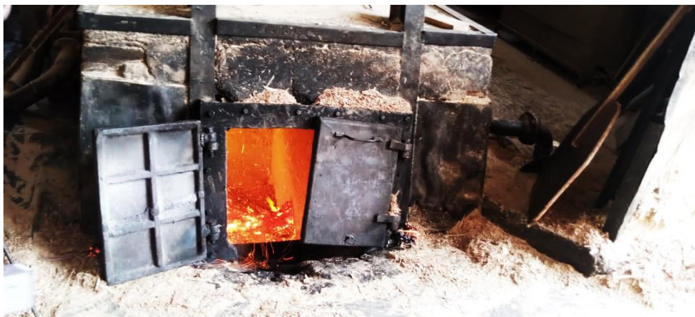
Waste as a fuel for the Boiler House( Source: Author's Construct,2023)
