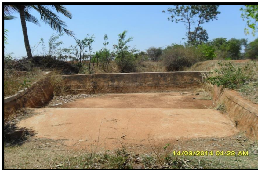
Picture – 1: Check dam in the Area (good one)
